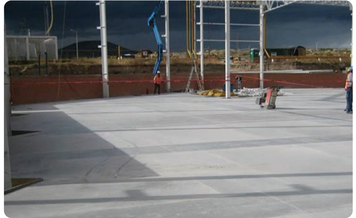
Industrial floor – OC Puma plant, Mexico. 10 kg/m 3 Anti-CRAK® HP 67/36 + 0.6 kg/m 3 Anti-CRAK® HD12, C 25/30
